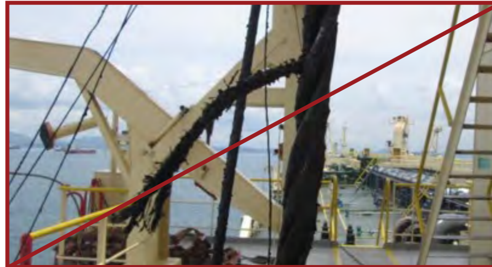
Lifeboat wire that will not pass inspection
