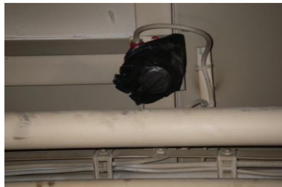
Smoke detector covered by plastic bag.
