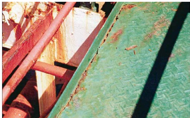
Catwalk cracked.
