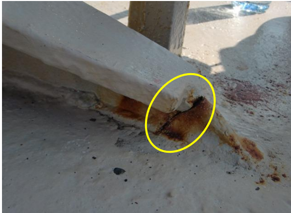
Cracked hatch coaming end bracket.
