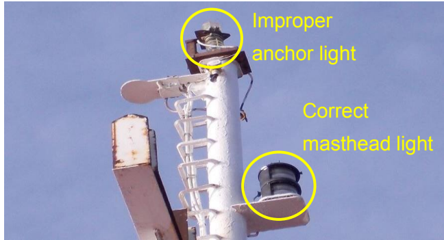
Signal light installed improperly as anchor light. Correct masthead light is to cover a 225 degree arc of the horizon.
