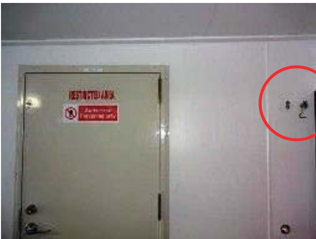
Unacceptable hold-back hook for door (required to be self-closing)!
