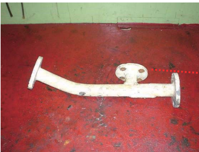
Flange connection to by-pass line
