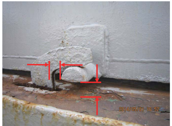
Excessive gaps of hatch cover
