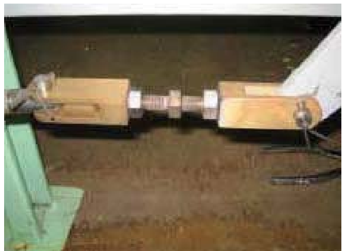
Correct condition of turn buckle
