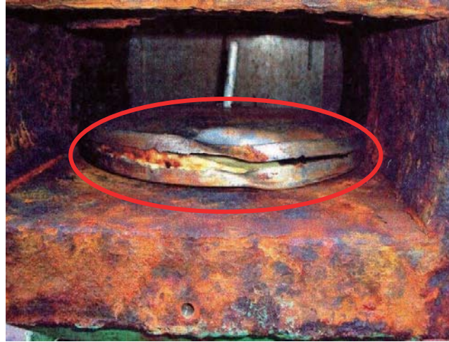
Damage of disk float
