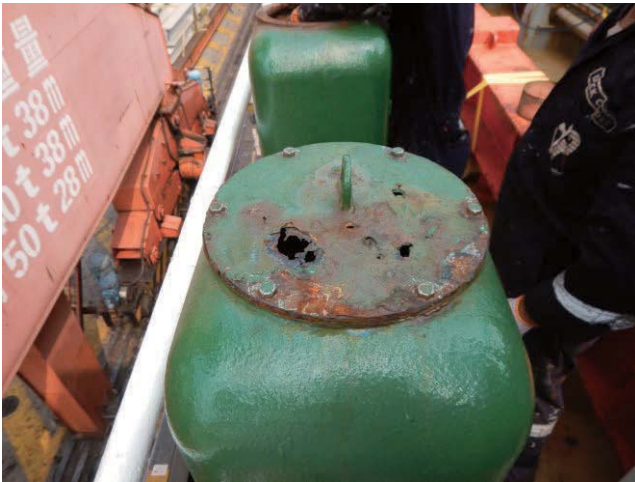
Corrosion holes in air pipe head
