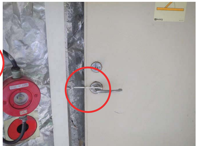
Unacceptable hold-back hook for door (required to be self-closing)!
