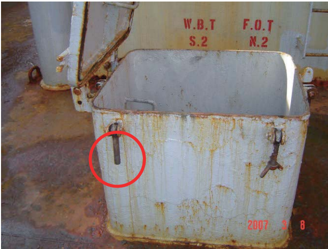
Missing nut of small hatch
