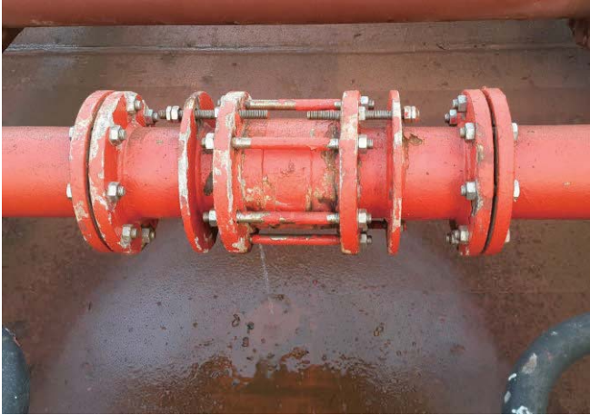
Leakage of fire line
