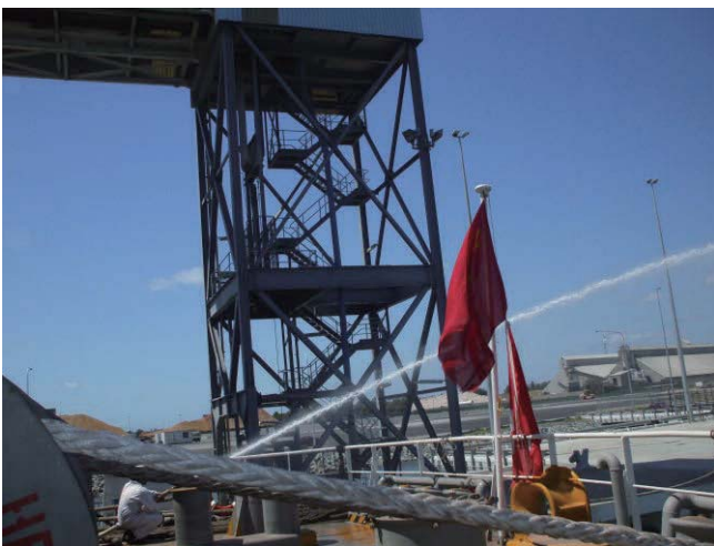
Performance test of emergency fire pump
